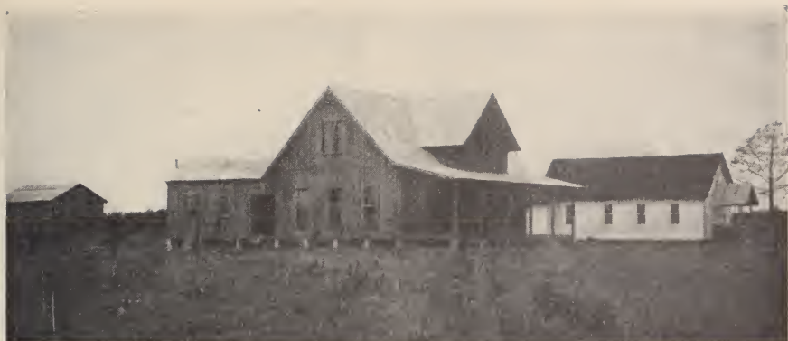
CHURCH AND RECTORY AT SANTA FE
